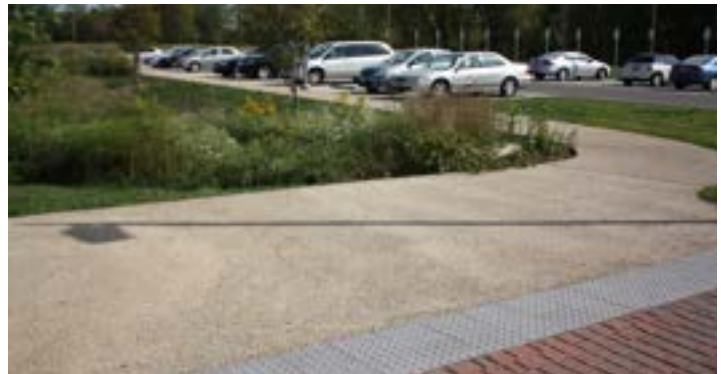
Example of porous pavement and a rain garden
