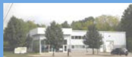
A renovated Nickles Bakery could be combined with the nearby West Michigan TV repair to create a secondary commercial cluster.
