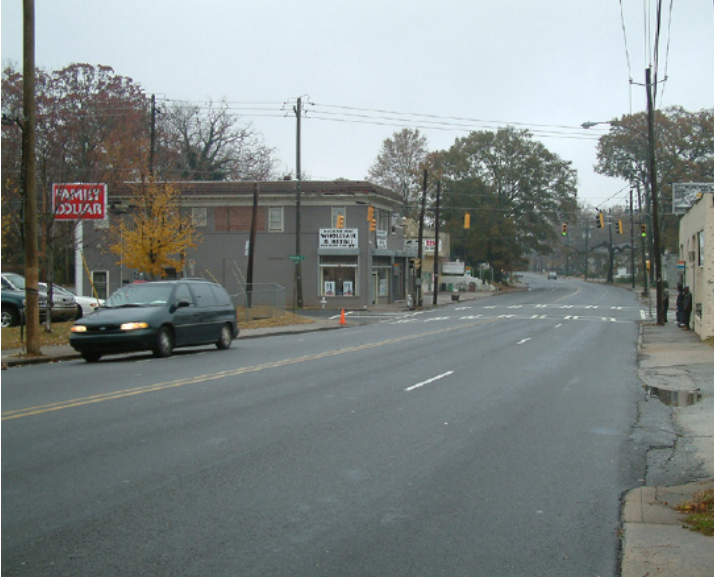
Atlanta's Cascade Avenue, with up to 17,900 vehicles per day, is a challenge to walk, bicycle or shop.
