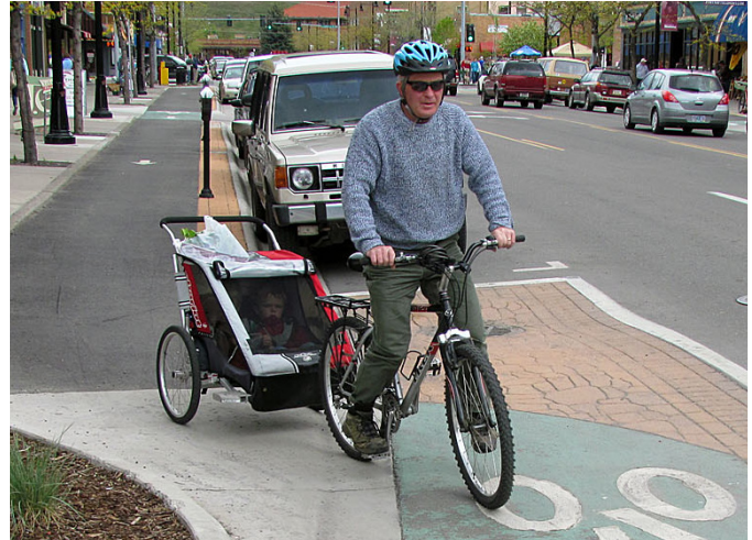
This raised cycle track in Missoula, Mont., is an example of a grade-separated, protected bike lane.
