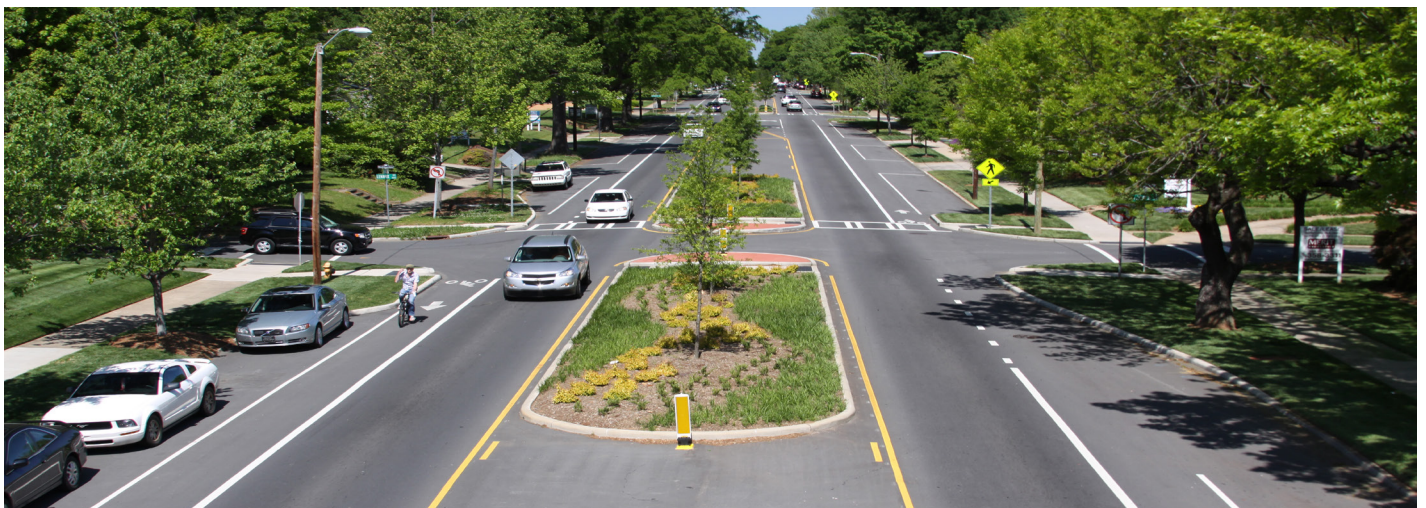
A road diet on East Boulevard in Charlotte, N.C., reduced travel speeds, bicycle and pedestrian injury rates and the number of rear-end and left-turn collisions. (Photo courtesy city of Charlotte)
