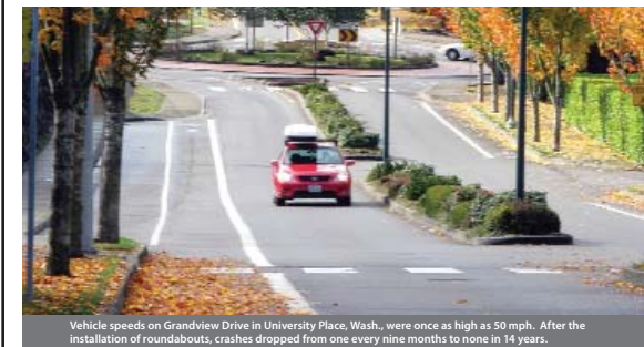
Vehicle speeds on Grandview Drive in University Place, Wash., were once as high as 50 mph. After the installation of roundabouts, crashes dropped from one every nine months to none in 14 years.
