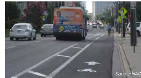
Buffered Bike Lane in Austin, TX
